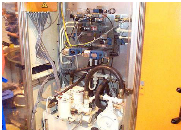
Fig. 33 Example: Valve test stand with 5-µm filtration
